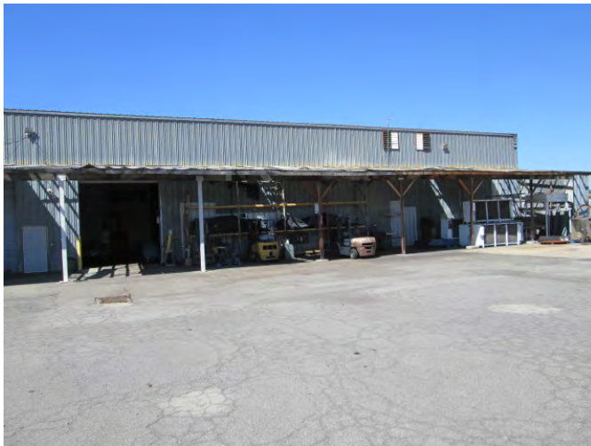
15. Western view of the eastern side of the warehouse building.
