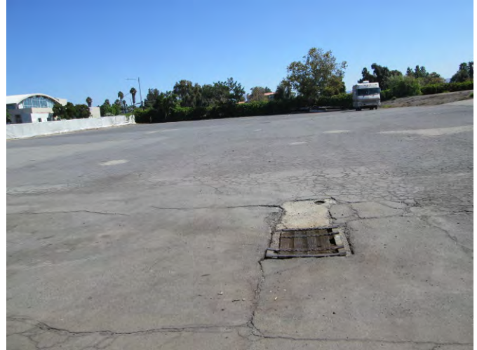
14. View of northeastern portion of the Site.
