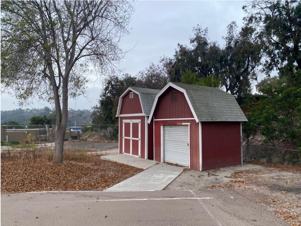
5. View south of Kindergarten storage sheds.
