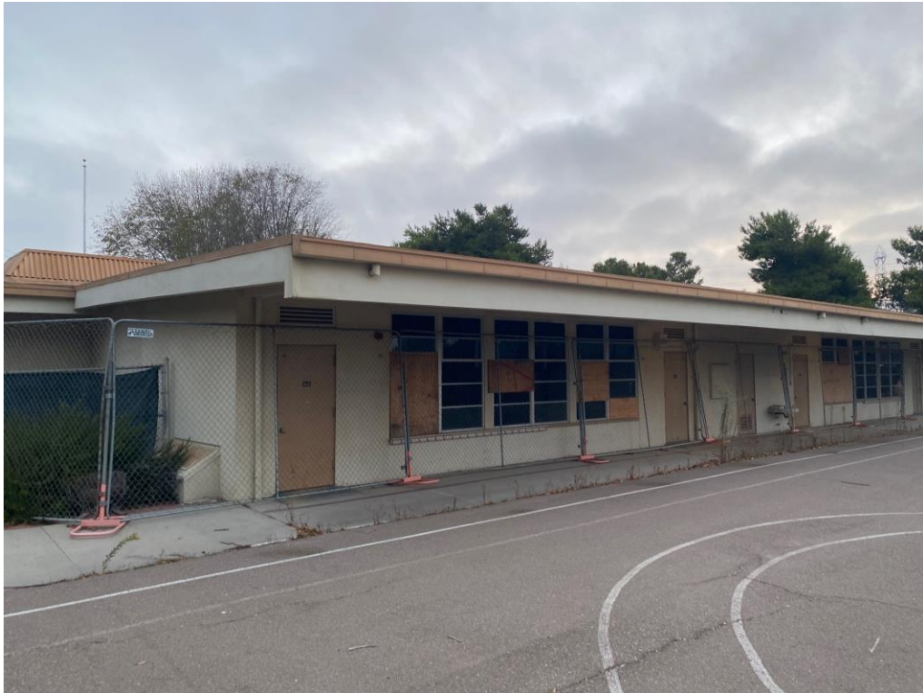
3. View south, of typical classroom building.
