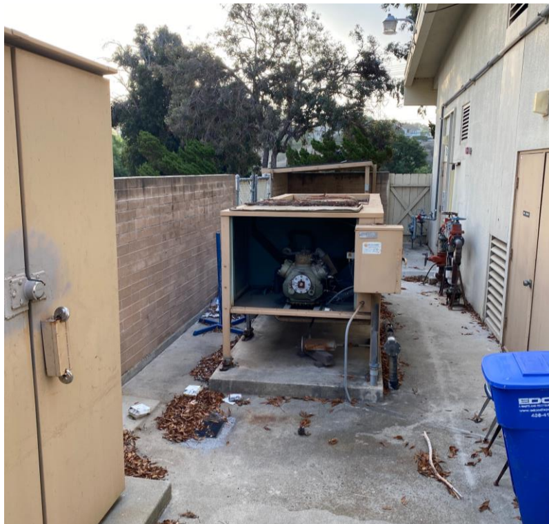
28. View eastward, of miscellaneous mechanical items.
