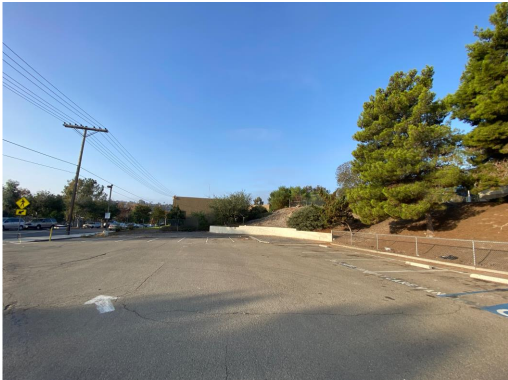
32. View south, of front parking lot drop-off area.
