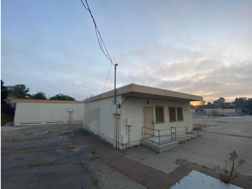
13. View north towards portable classrooms near asphalt playground.
