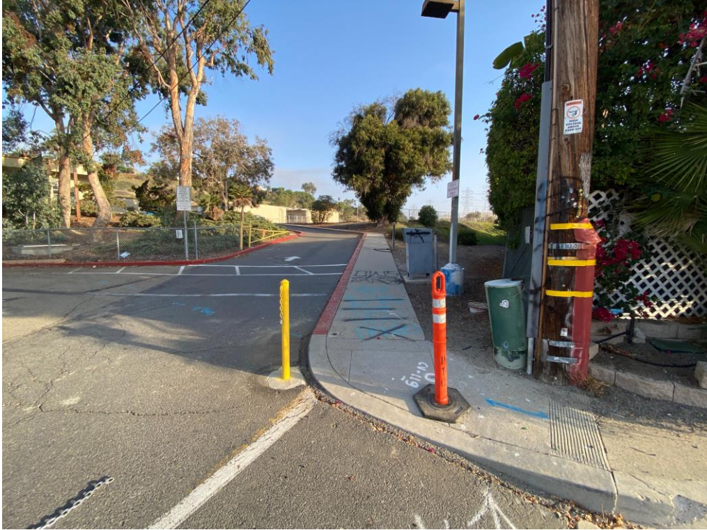
31. View northwest, of driveway.
