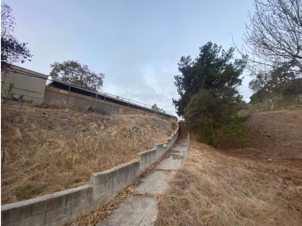
9. View west towards La Cresta Drive Multi-Family Residential covered parking.
