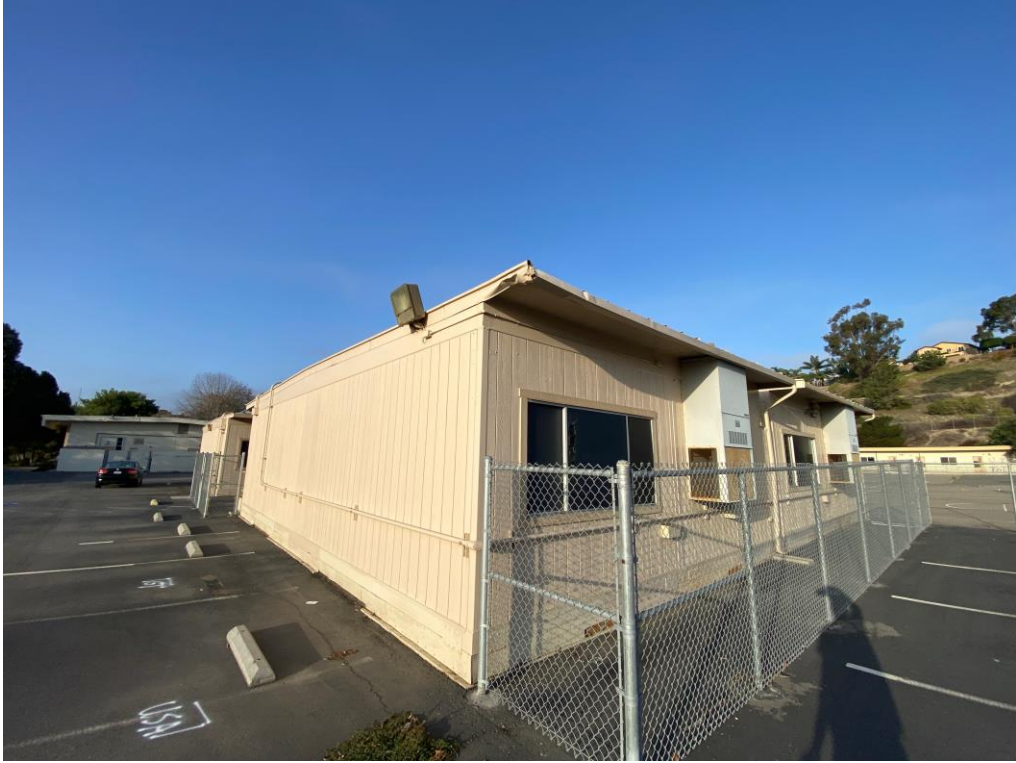
29. View of portable classrooms.
