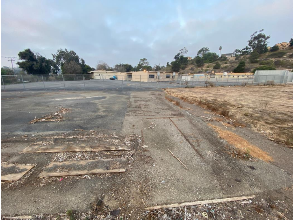
23. View south, of previously existing structure.
