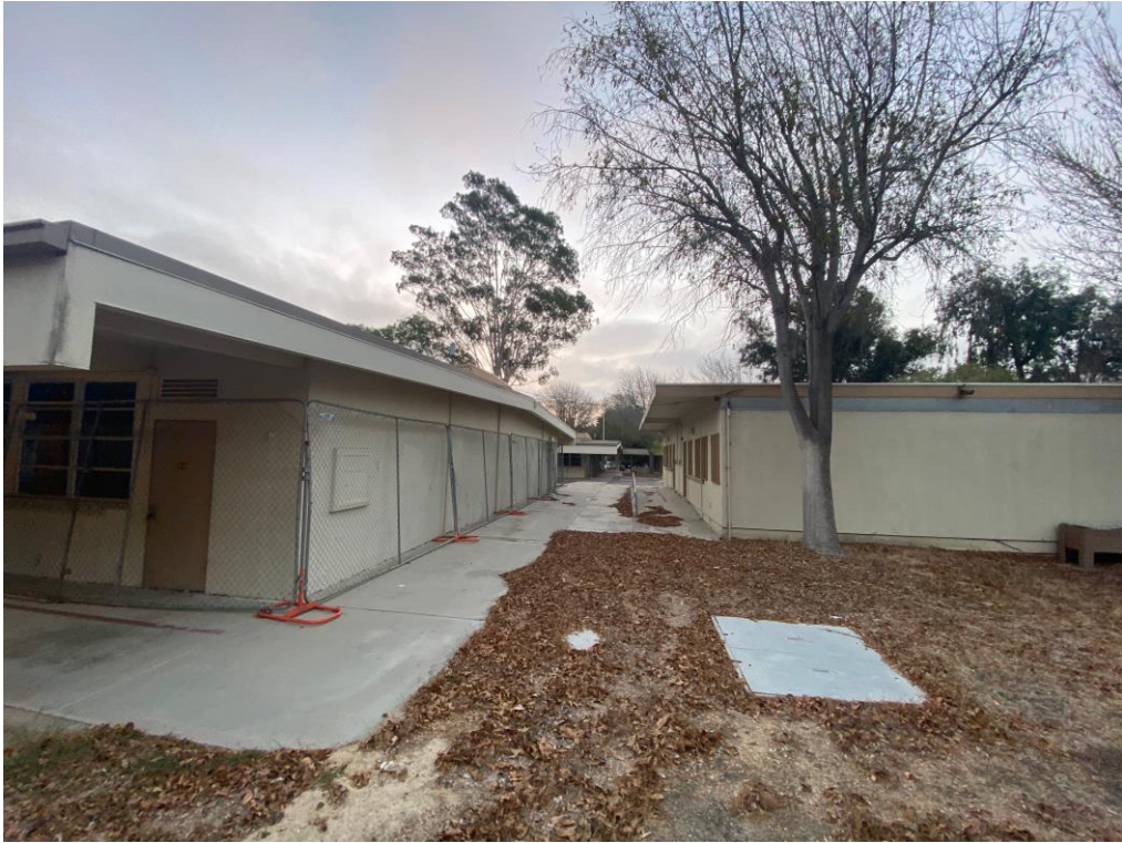
11. View east towards typical classroom and Staff Lounge/Library building.
