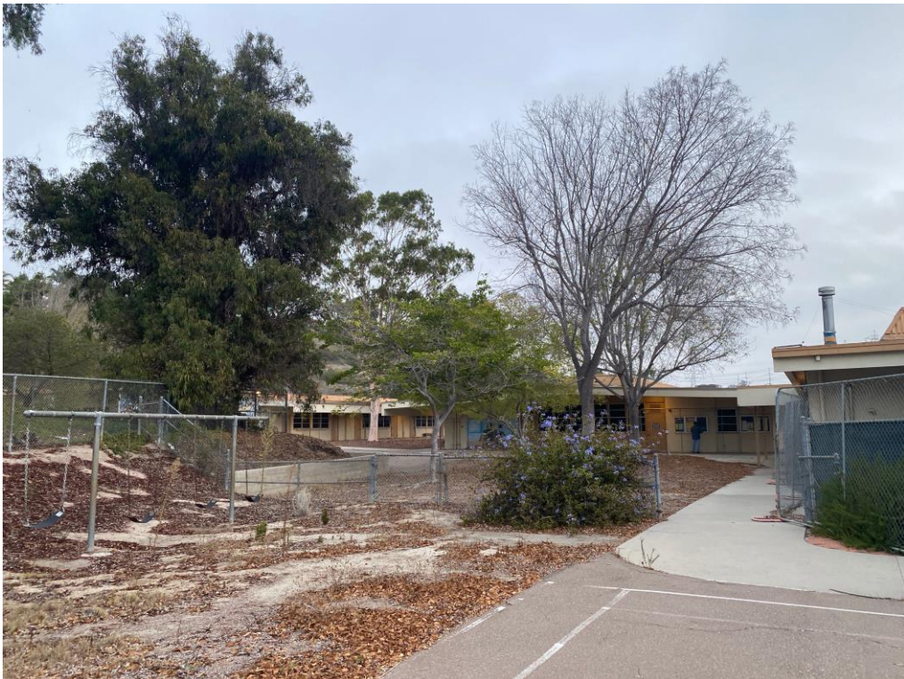
6. View north from Kindergarten playground towards classrooms.
