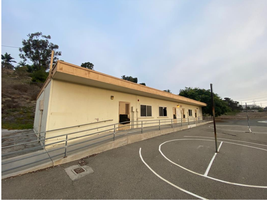
27. View northwest, of portable classrooms.
